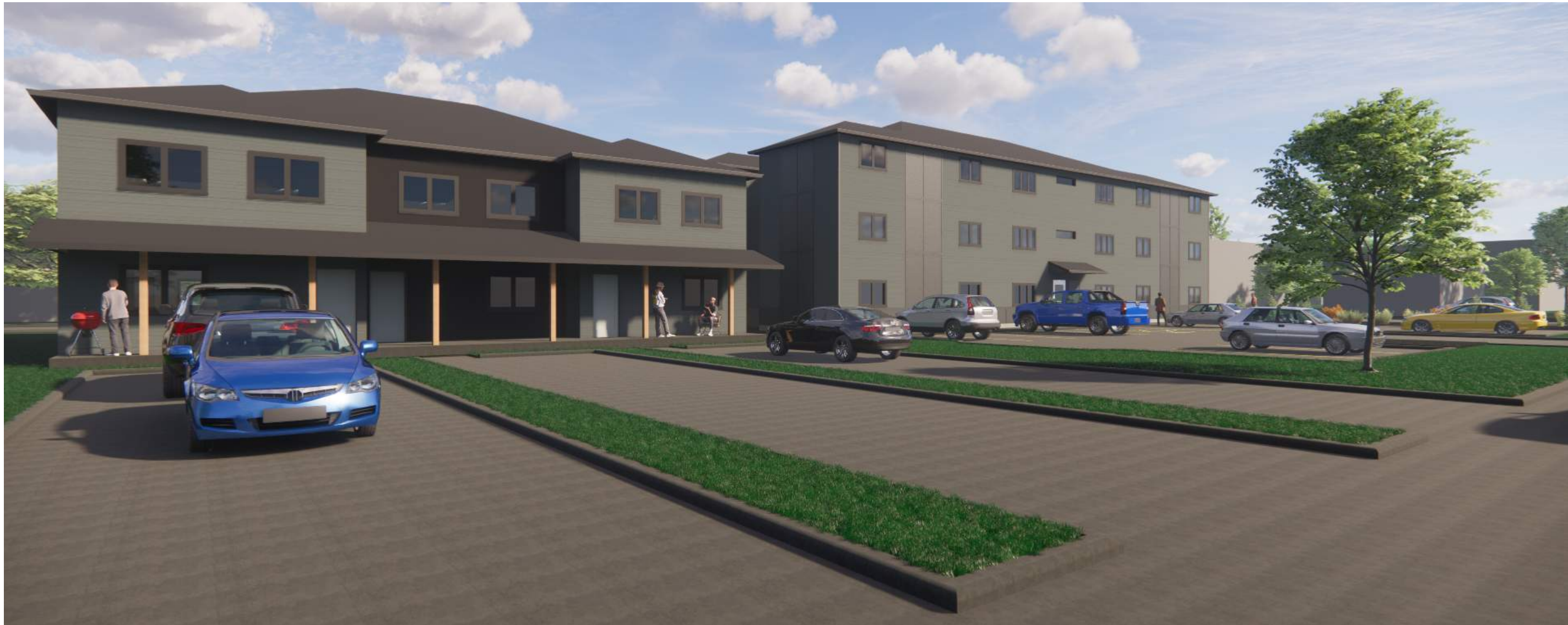
LOOKING TO THE SOUTHWEST FROM THE ALLEY AT BOTH BUILDINGS
