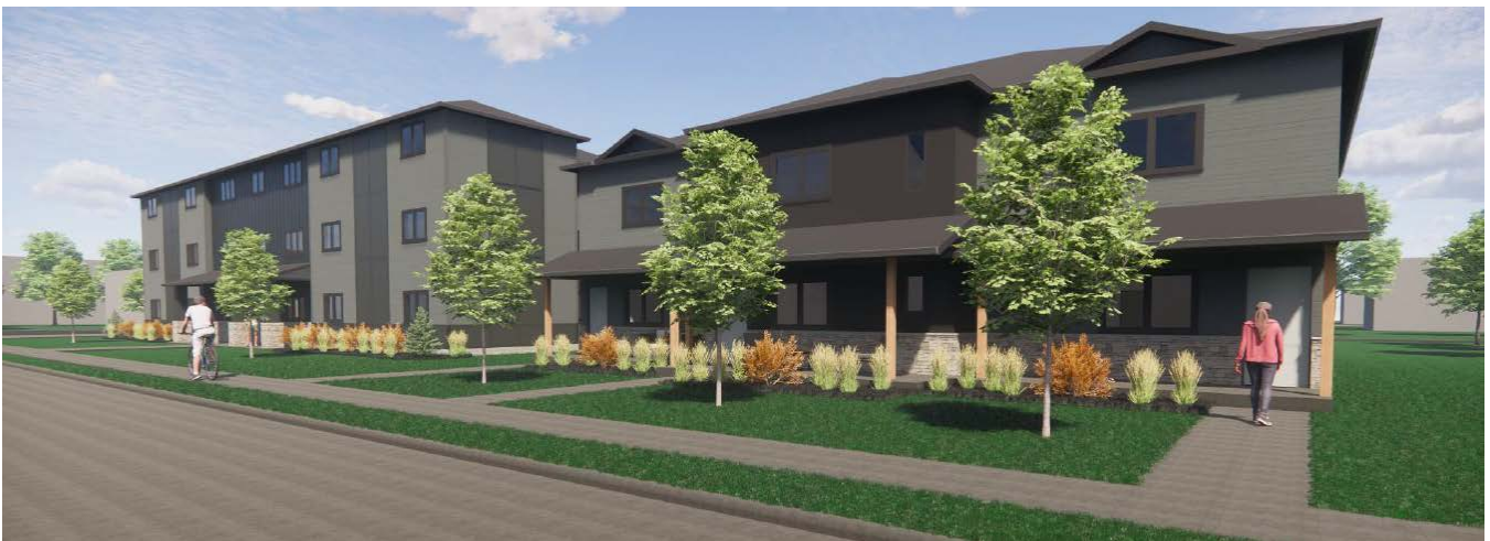
Looking to the northwest from Starr Street
