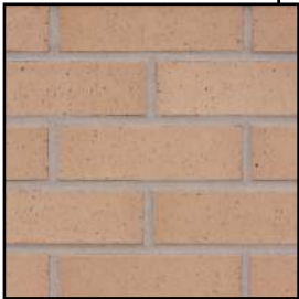
Face Brick Modular Running Bond
