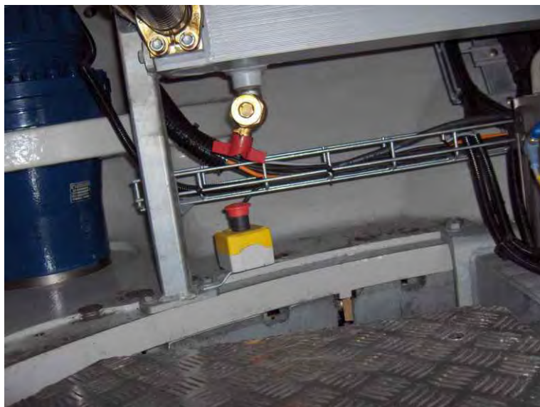
Picture 2 Yaw ring emergency stop button (pos. 2, Figure 1)
