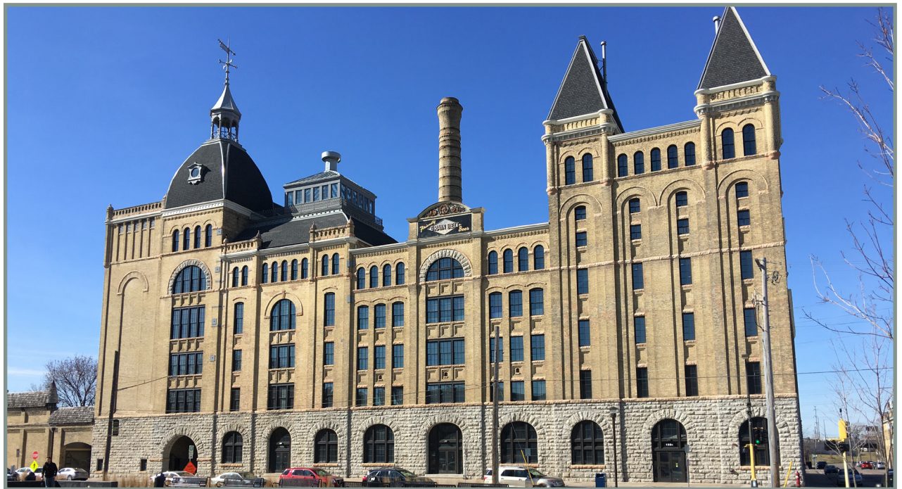
The synthetic slate roof on the Grainbelt Brewery in Minneapolis is nearly identical to the original slate roof given the height and scale of the building.
