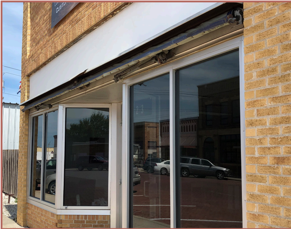
The above storefront has a modern aluminum frame with the original roller awning intact above. The unpainted metal stands out from the buff brick facade and is not a recommended replacement.
