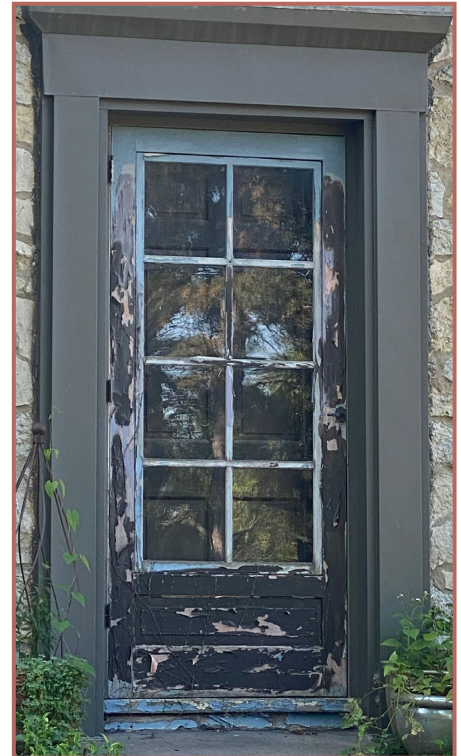
Modern full light storm door with concealed screen (left) and historic 8 lite storm door which needs maintenance to maintain its operability (right)
