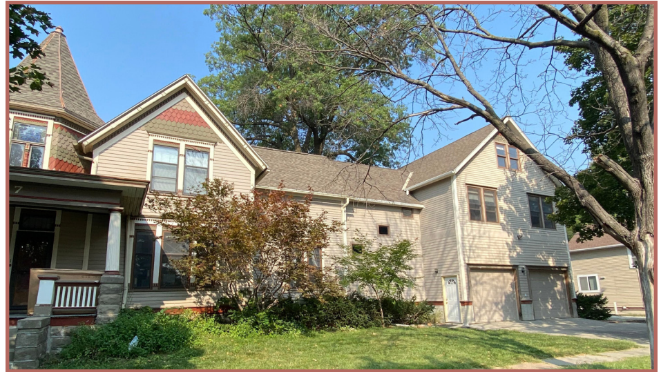
The two story link with three story garage addition competes with the original home in overall scale and massing, however the neutral color palate and matching roof pitch with step back in the link portion are in alignment with the historic home.
