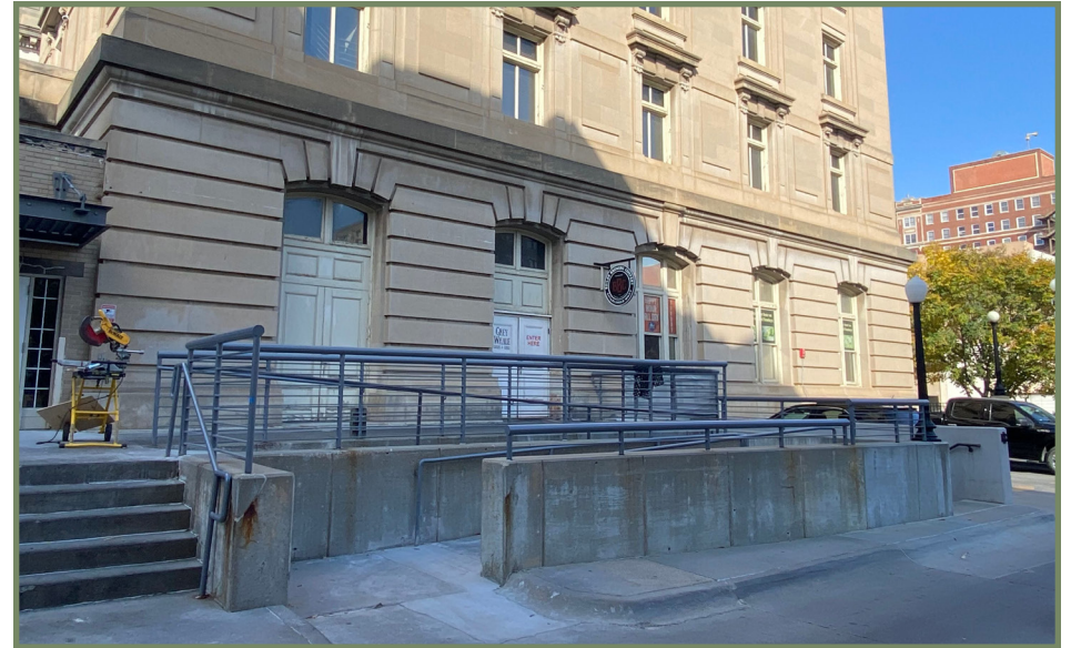
The image above shows the Old Federal Building with a ramp added to the rear of the building. The grey color of the railing does not compete with the building, however the amount of rails starts to interfere with the facade. It's location on the rear is ideal for a treatment of this level.
