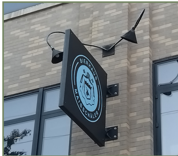
The image above shows gooseneck lighting to illuminate the sign with indirect lighting.
