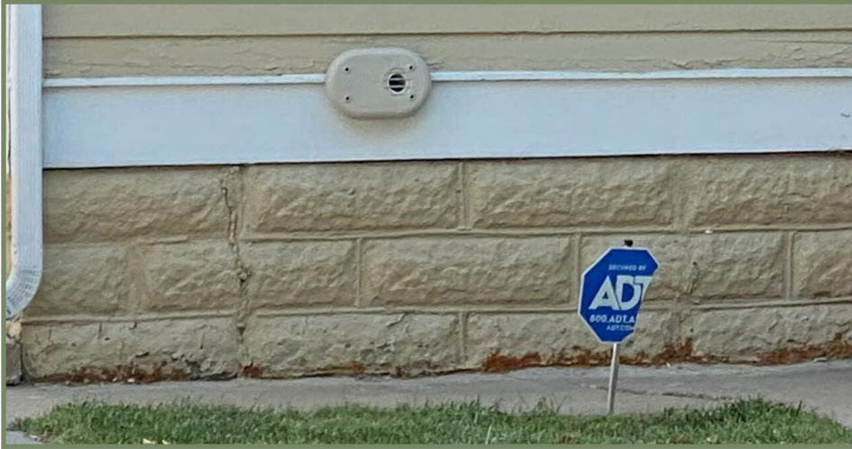
Historic rock-faced concrete block foundation that should be retained for either structural reuse or aesthetic reuse.
