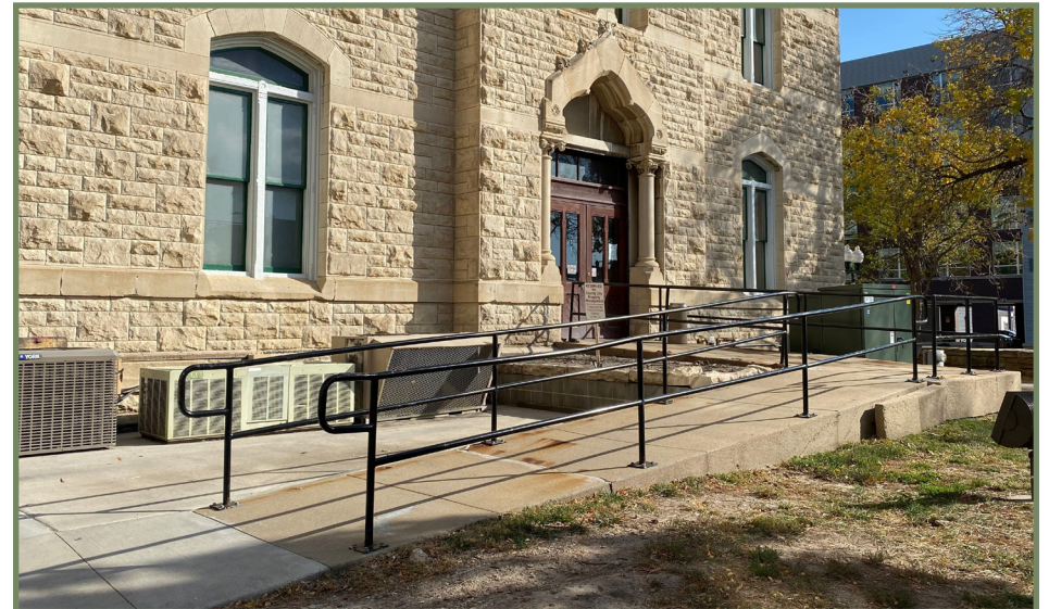
The image above shows the Old City Hall with a ramp added on the side with a simple black railing that does not obscure the facade.
