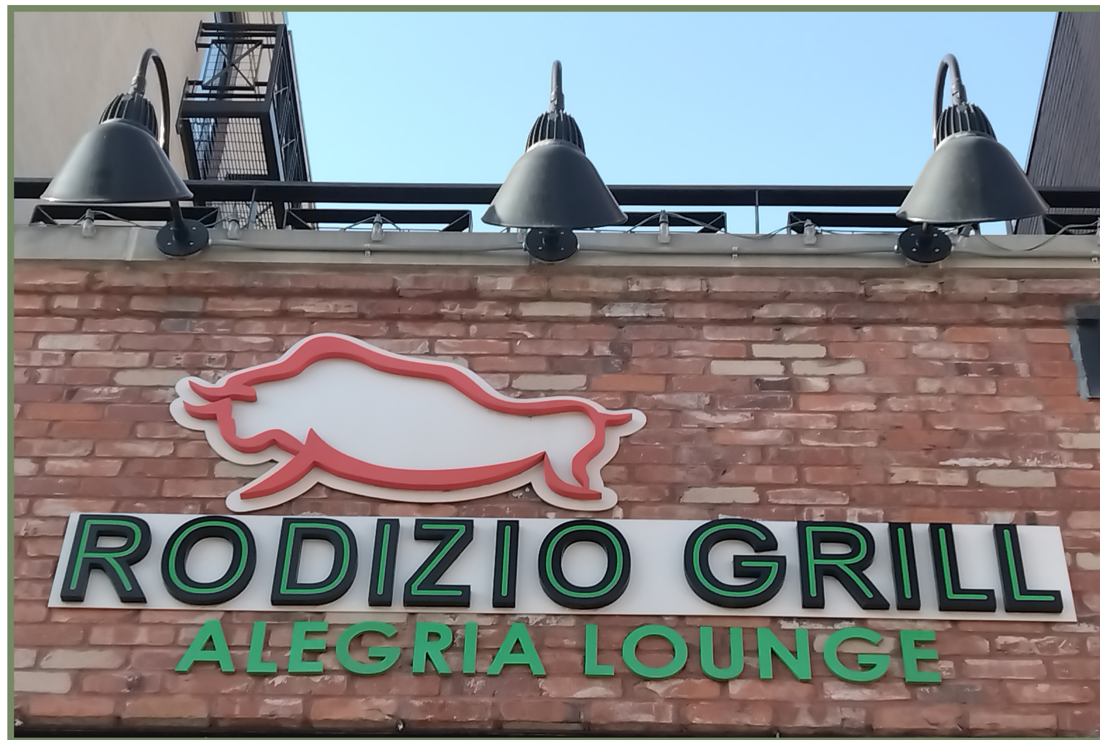
The wall sign is scaled to fit below the corbeled brick cornice and does not compete with the architecture of the building.
