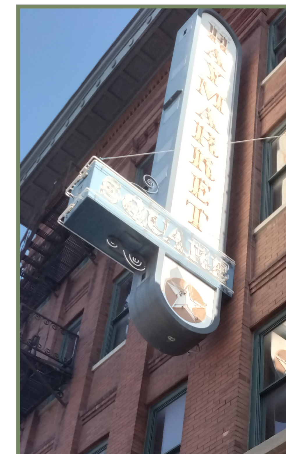
Projecting sign identifying the building which is positioned in the center of a pilaster.
