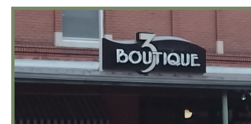
Shown above is an example of signage mounted above the canopy, but within the edges.
