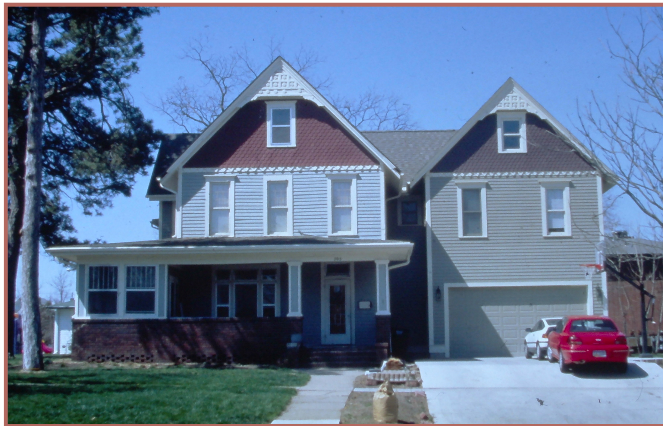
The addition to this home for the garage has similar results as above, also with the problem of a modern garage competing with the main porch and entrance to the home given the close proximity.
