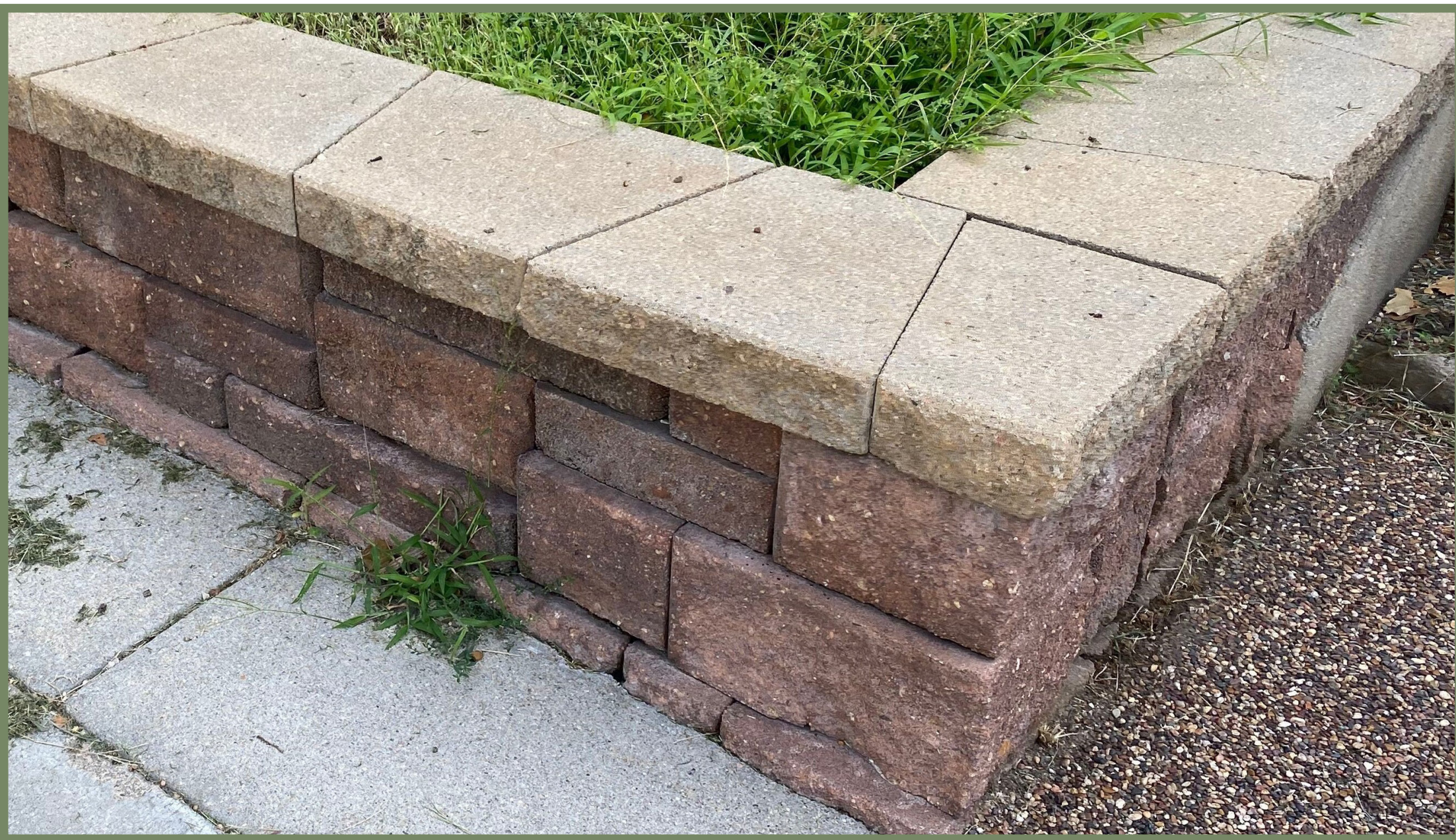
A low masonry wall finished with a cap to stabilize the yard.
