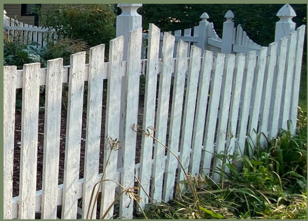
Example of a fence less than 48 inches in height with greater than 50 percent opacity.
