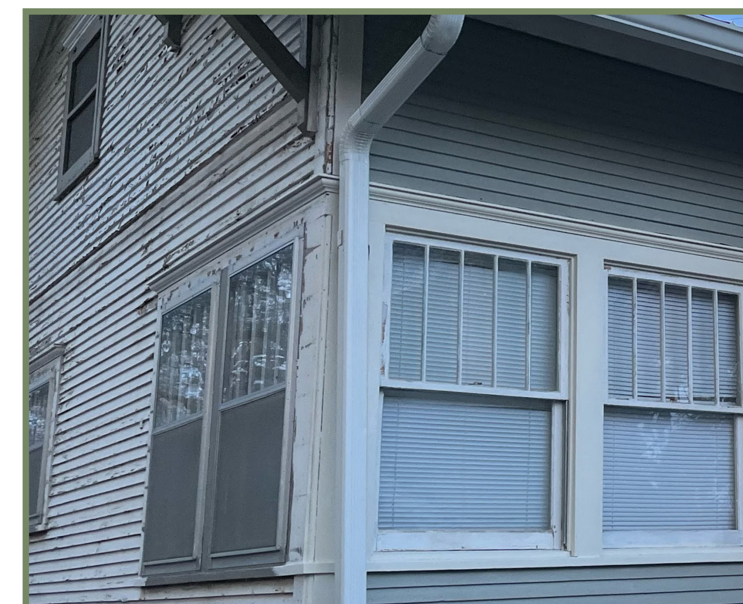
The images above show the progress of removing vinyl siding that damaged the clapboard siding and caused the removal of window surrounds which needed to be rebuilt and patched. The picture on the right shows the front finished elevation, newly painted, with a side elevation relieved of the vinyl siding awaiting a fresh coat of paint.
