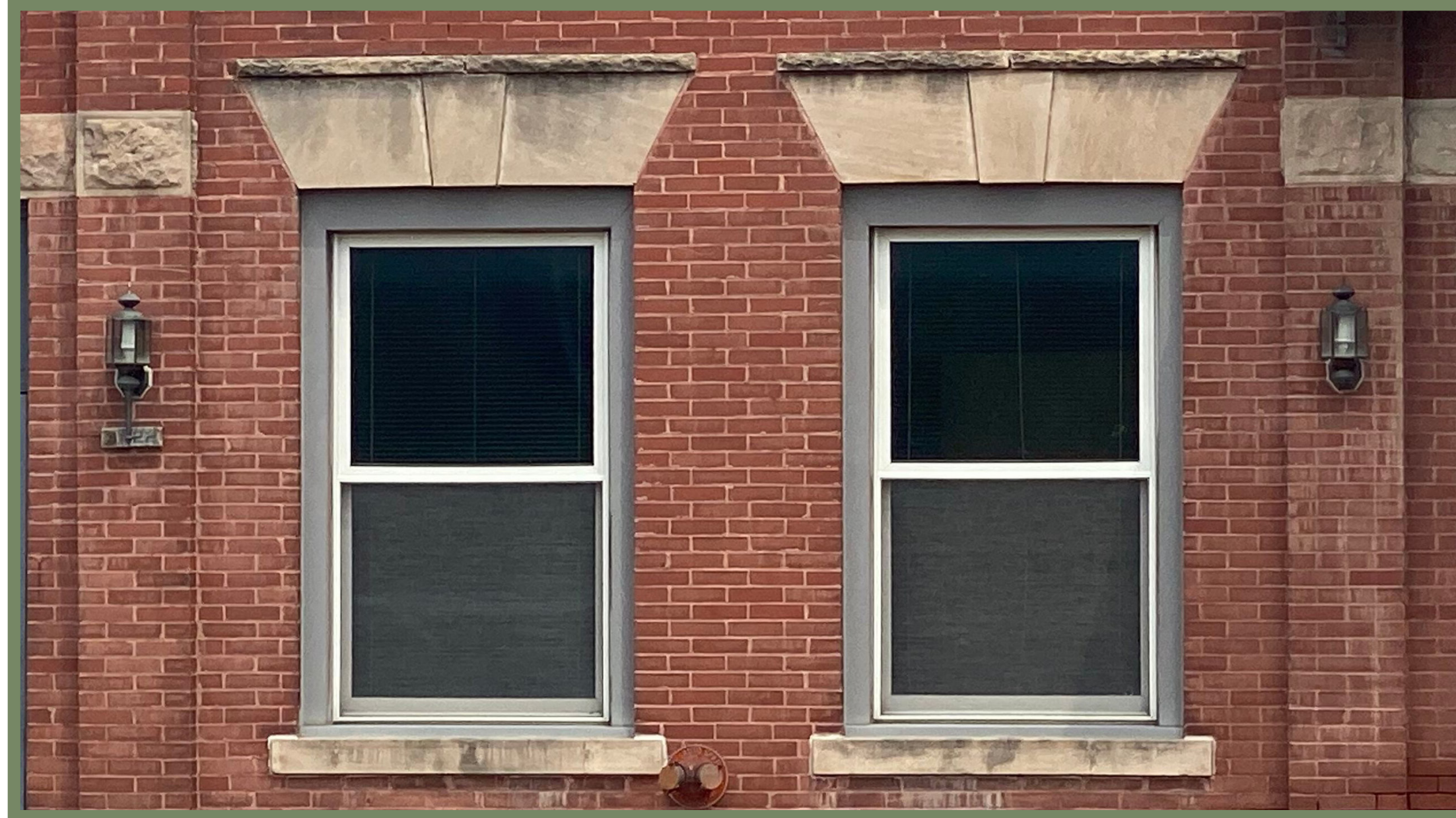
Wall sconces installed in the first floor pilasters are scaled appropriately and fit the period of the historic architecture.
