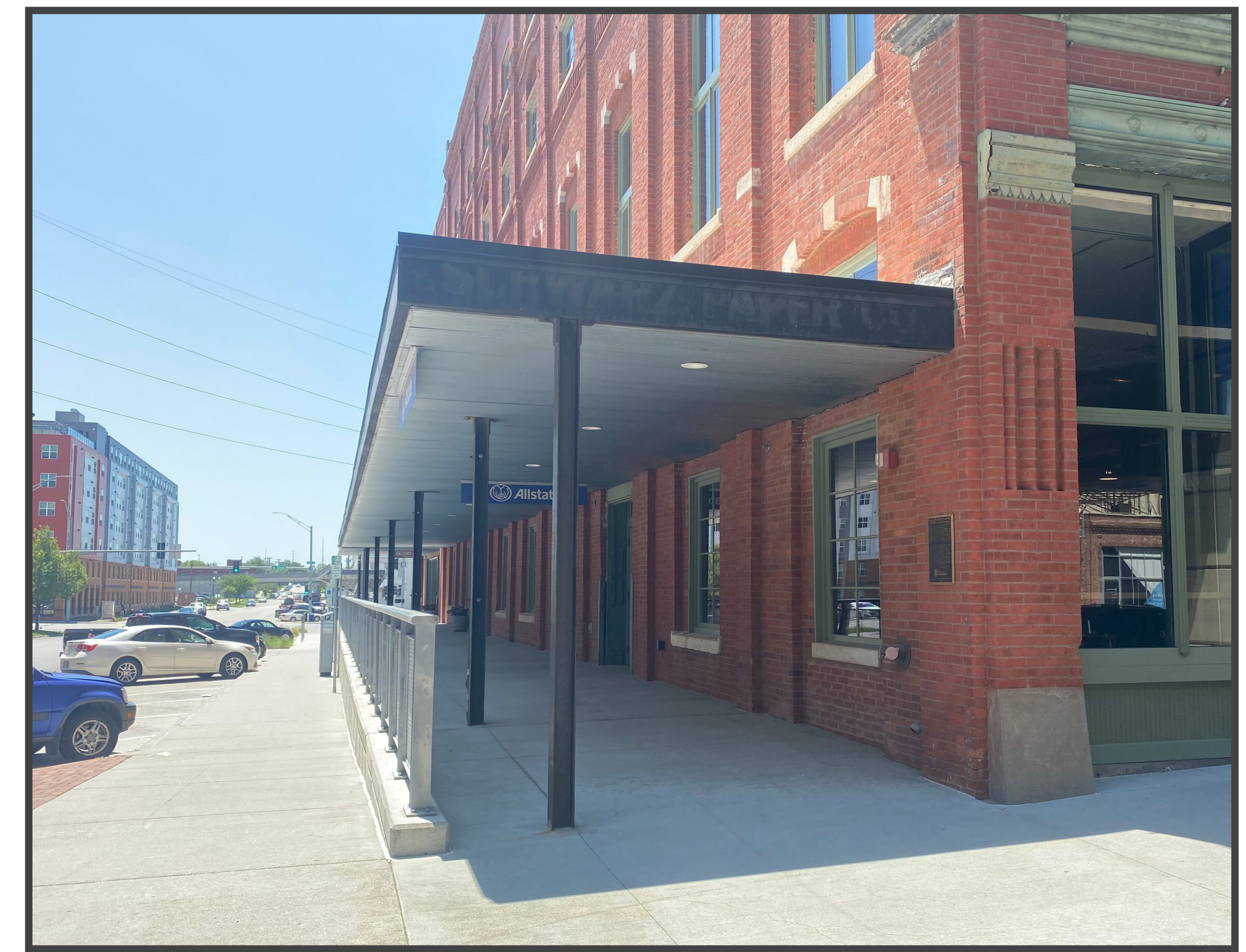
Post supported canopy
