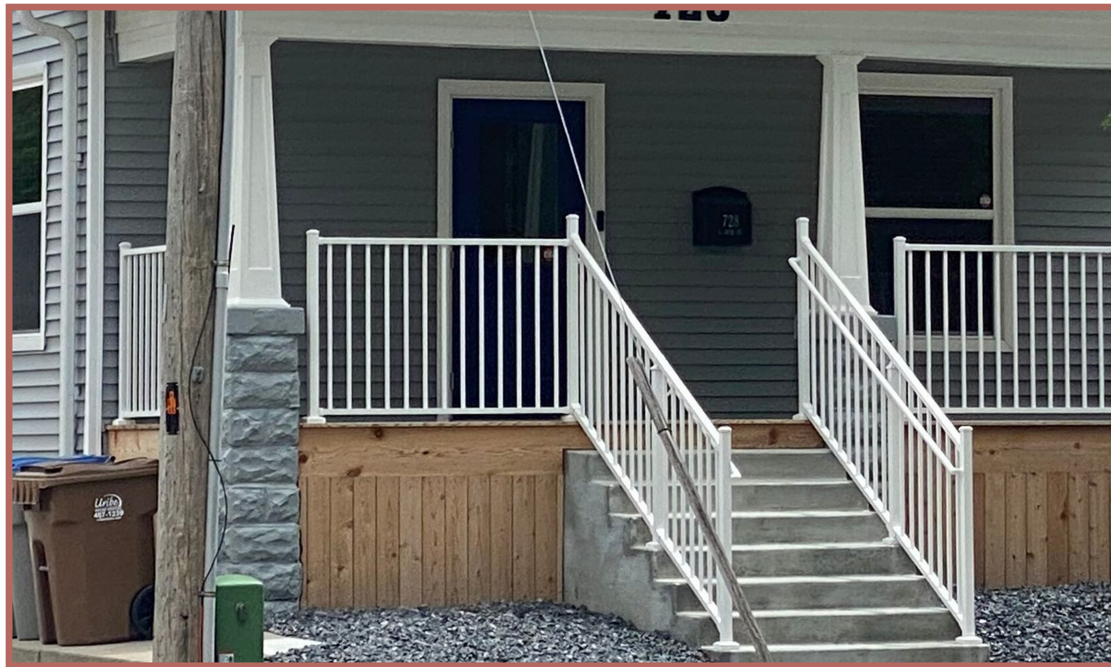
The porch skirting and railings above are not an appropriate treatment for a historic building. The square columns that replaced originally rounded columns illustrate the panel design with base and cap concept, however the tapered design is not true to the prairie box style of the home.
