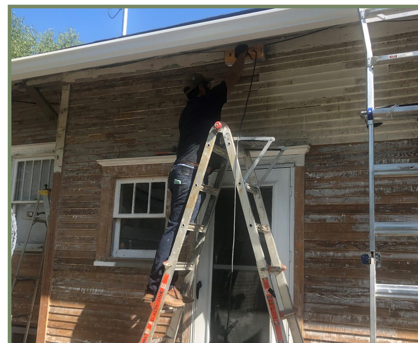
The images above show the progress of removing vinyl siding that damaged the clapboard siding and caused the removal of window surrounds which needed to be rebuilt and patched. The picture on the right shows the front finished elevation, newly painted, with a side elevation relieved of the vinyl siding awaiting a fresh coat of paint.
