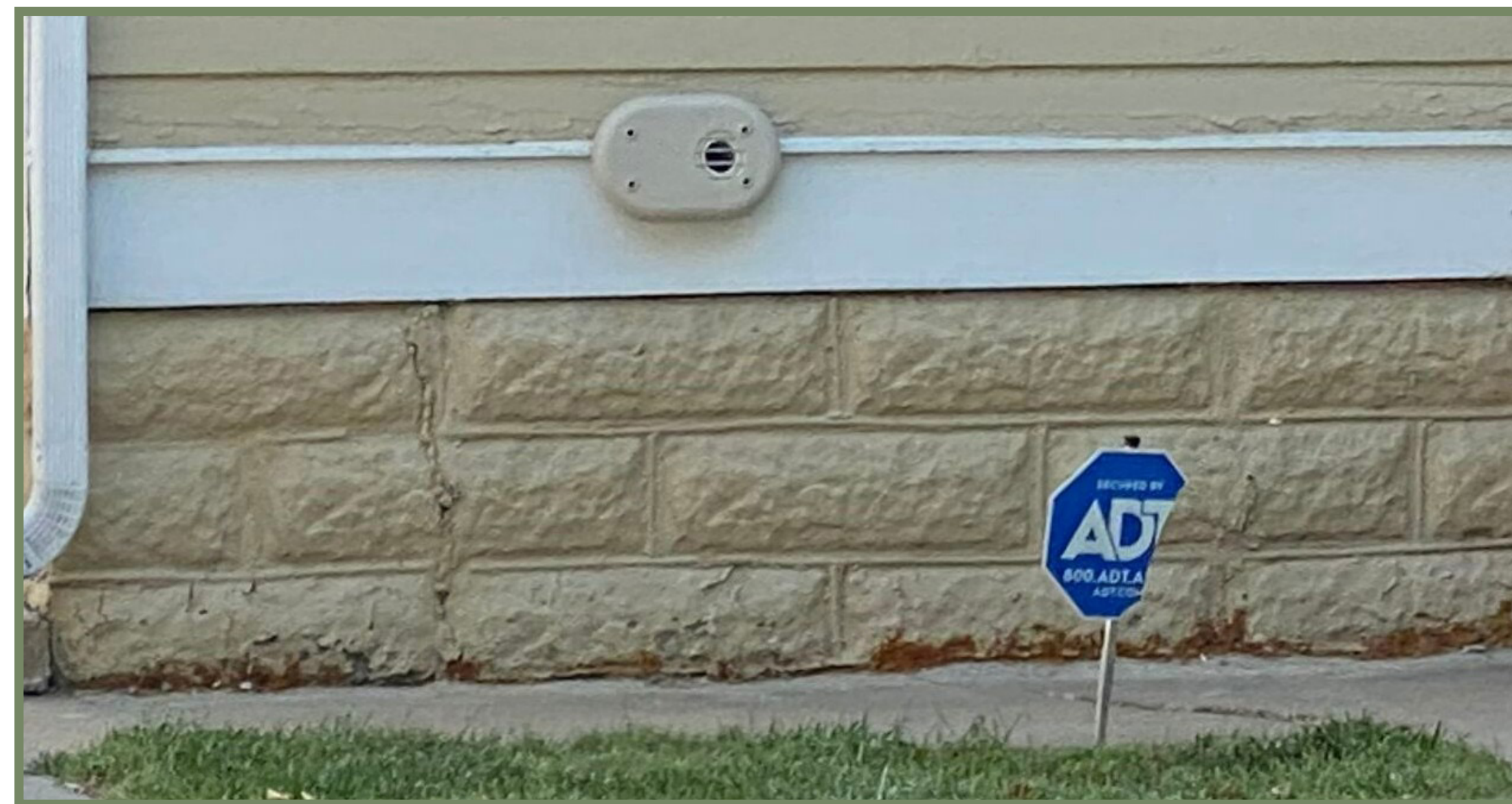
Historic rock-faced concrete block foundation that should be retained for either structural reuse or aesthetic reuse.
