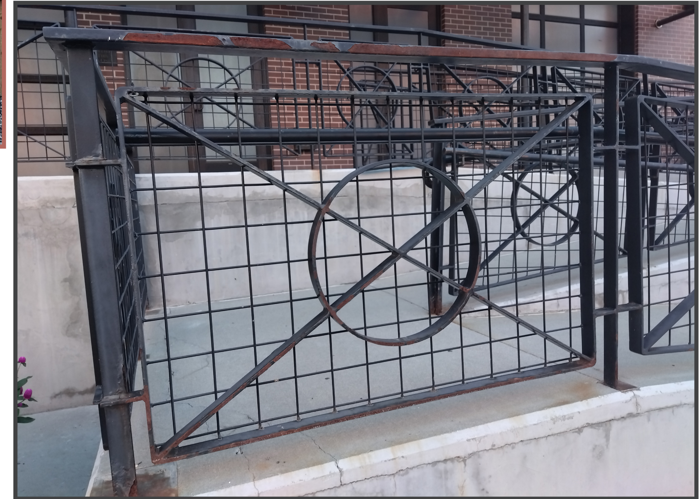
Dock railing example commonly found in the Haymarket Historic District with a simplified design. Given the rust showing, the metal type used on future projects should be looked at for compliance with the guidelines.
