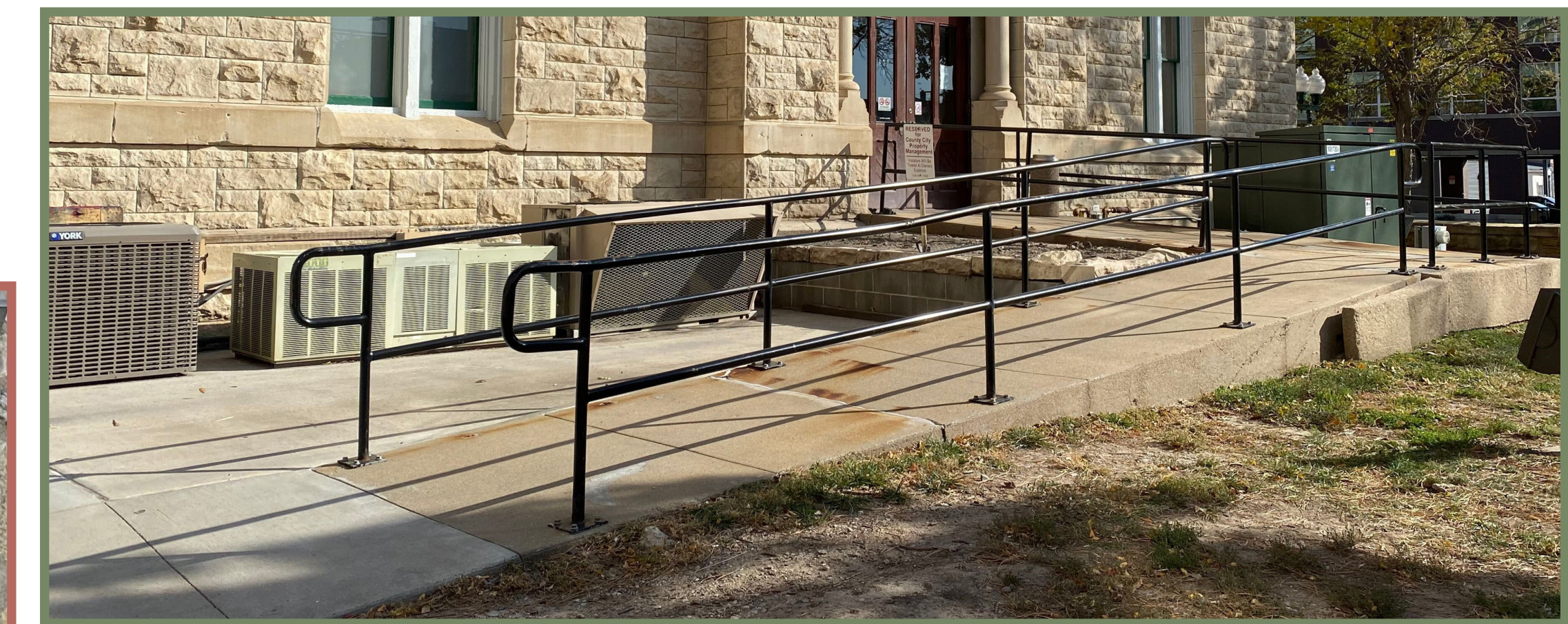
The image above shows the Old City Hall with a ramp added on the side with a simple black railing that does not obscure the facade.
