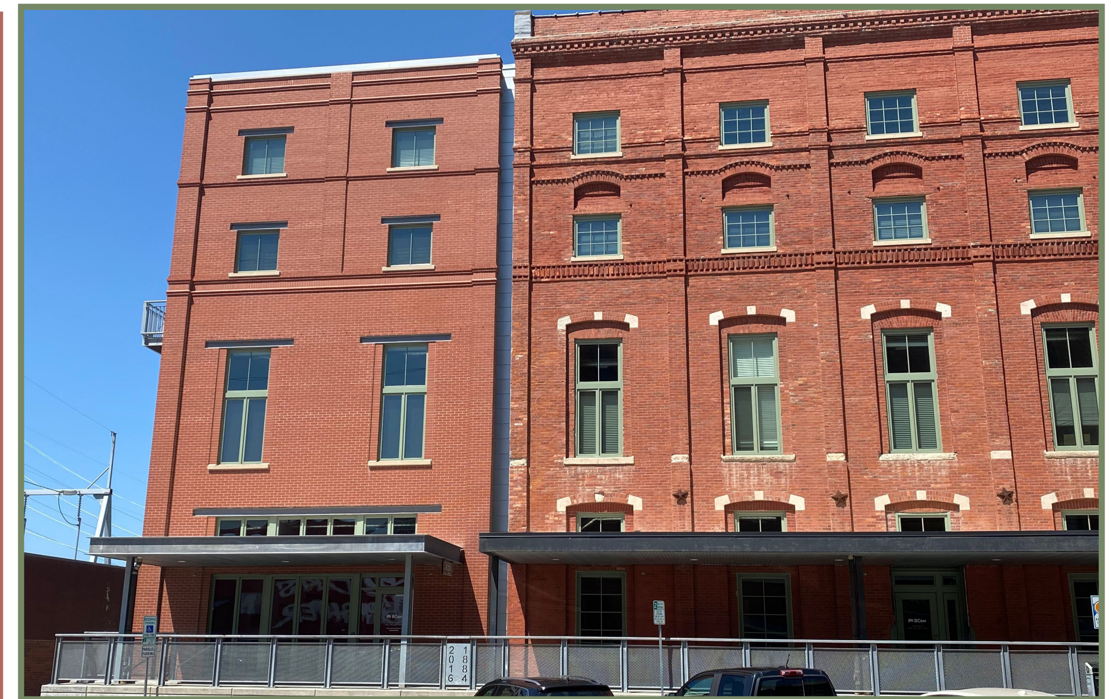
The addition (left) to the Sullivan Building is located at the rear and reflects the character of the original structure in a simplified version of the intricate design.
