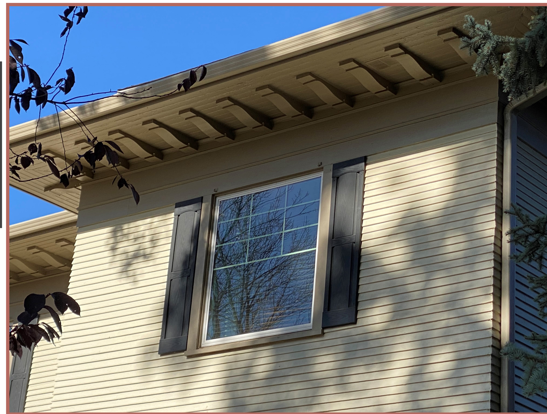
Flat look created with an applied muntin which does not replicate an original wood window divided light.
