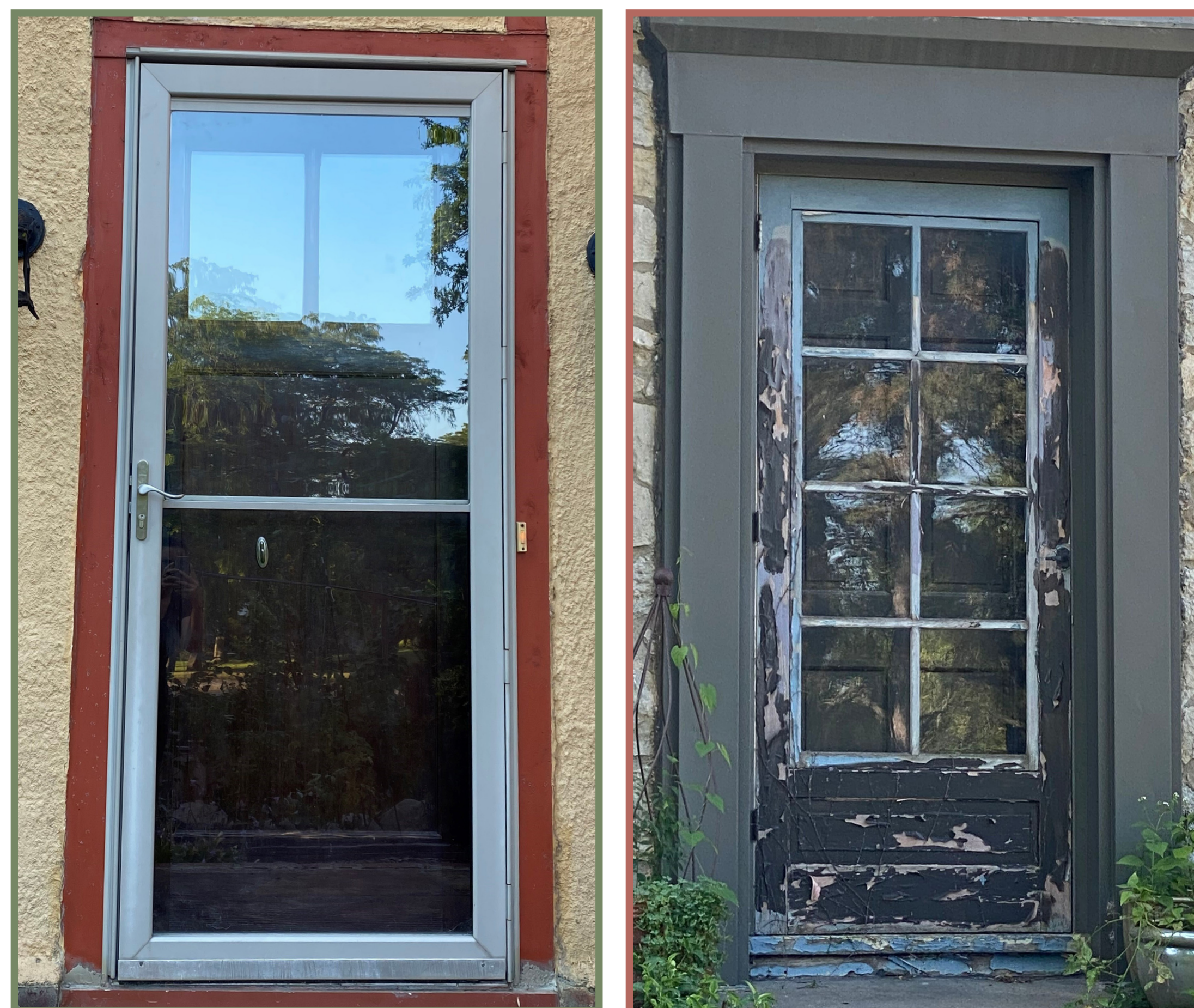
Modern full light storm door with concealed screen (left) and historic 8 lite storm door which needs maintenance to maintain its operability (right)
