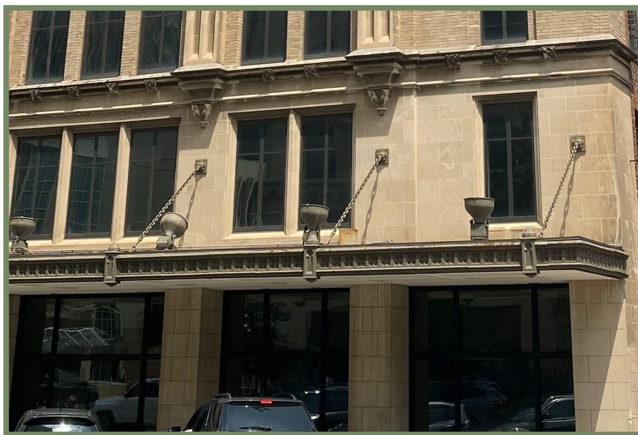
The above facade lighting mounted to the top of the canopy is appropriate for the historic commercial building, with an attempt to conceal their presence by painting them a similar color to the canopy.
