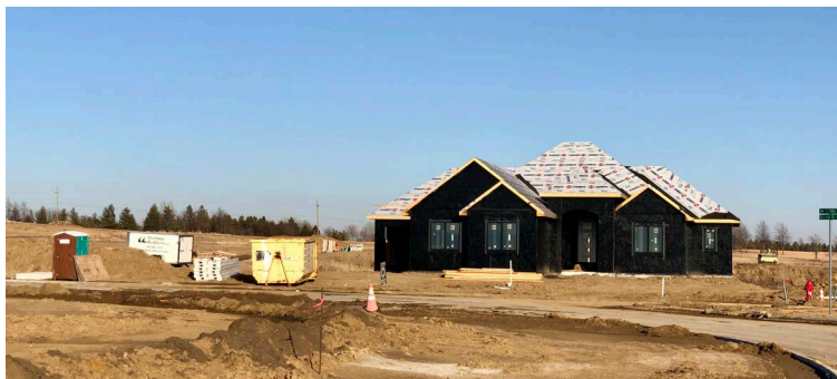
Home construction and site preparation near 93rd & A.
