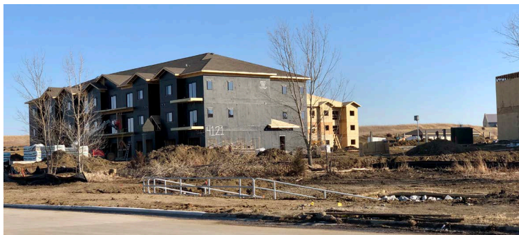
Traditional apartment complex under construction near 38th & Hohensee.
