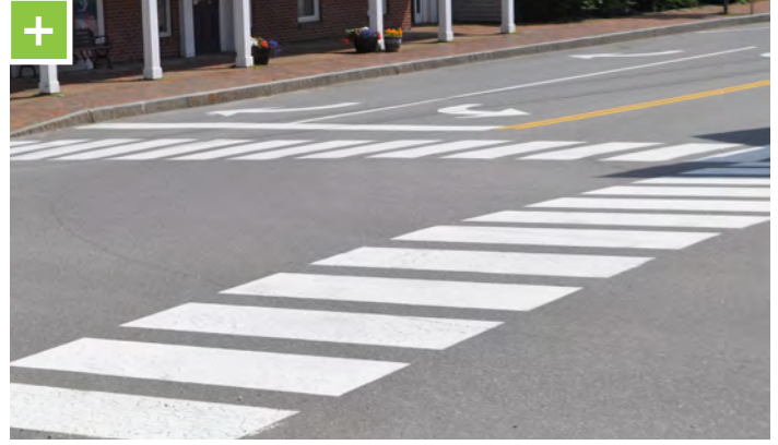
High visibility ladder crosswalks are more visible to all road users compared to standard crosswalks.
