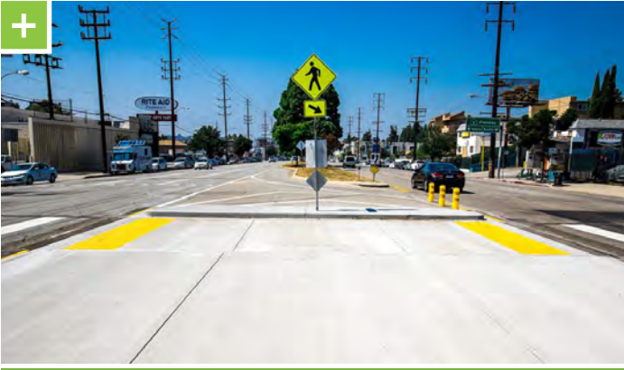
A long and wide pedestrian refuge island provides adequate space for pedestrians to wait for vehicular traffic to clear.
