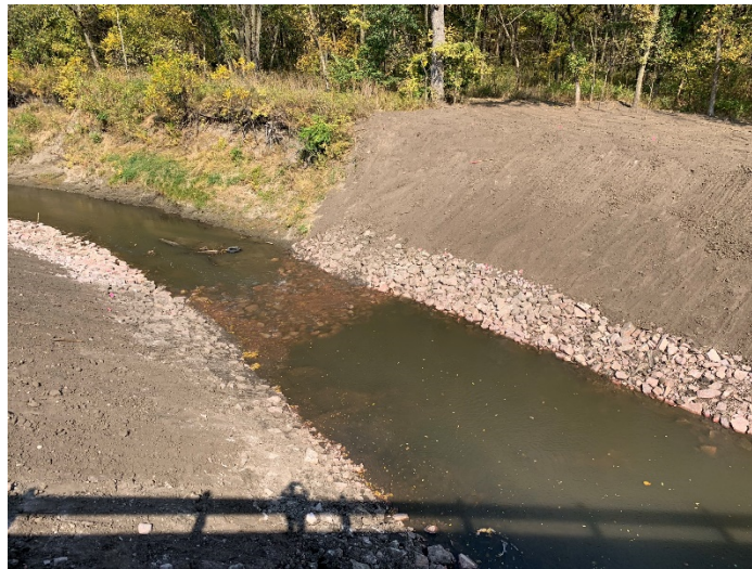
Example of Installed Grade Control
