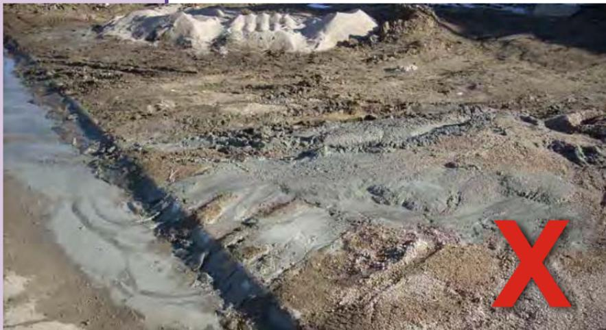
Each development should have designated concrete washout areas. If none exist contact the developer. The photo below is one example of a concrete washout area. There are many variations and designs for concrete washout areas. If maintenance is needed contact the developer. Never wash concrete into the storm drain.
