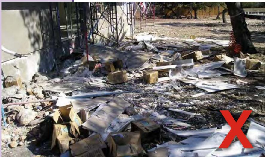
This is a combination of scrap drywall, drywall compound slurry, and other solid waste. The drywall slurry is considered a chemical spill, which is a violation.
