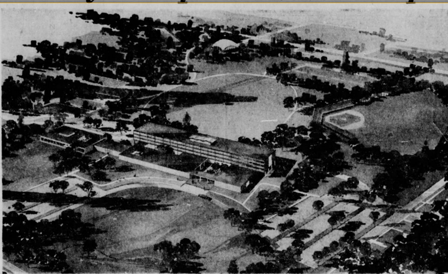
PROPOSED ROGERS TRACT COMBINED PARK-MEDICAL CENTER DEVELOPMENT —Architect's impression of how 300-bed Lincoln Medical Center (at center) and one-story Lincoln Rehabilitation Center and Handicapped School (left) might be situated on Rogers Tract so Park and Center complement each development without interference. Upper left corner is 33rd & O, looking to northeast. Proposed plan contains decorative park (upper left), swimming pool (top near center), recreation building (top at center), park lawn with several informal playing fields (above building), tennis courts (top right), informal, unlighted baseball field (right), reflecting pool and skating area (bottom), and off-street planted parking areas scattered around periphery. Hospital is sound-insulated by site arrangement, closed-window air control. Architect: Davis & Wilson, Associates Clark & Enerson.
