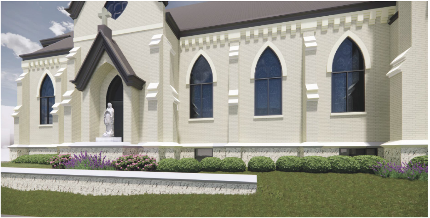
The renovation work underway at St. Mary's Catholic Church will help to preserve one of the Capitol Environs District's most iconic pieces of architecture.
