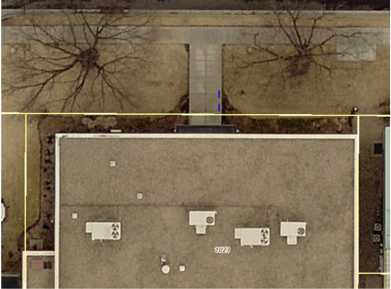
Rack locations in blue above on 10-foot-wide sidewalk leading to entrance.
