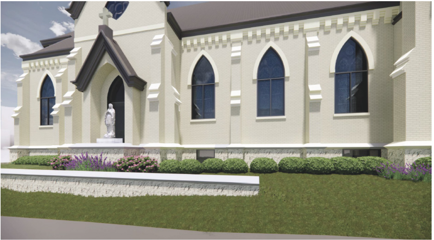
The renovation work underway at St. Mary's Catholic Church will help to preserve one of the Capitol Environs District's most iconic pieces of architecture.
