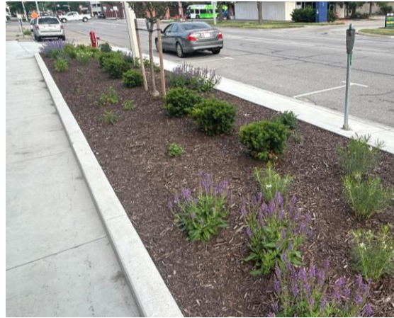
concrete planter curb – 14 TH St.
