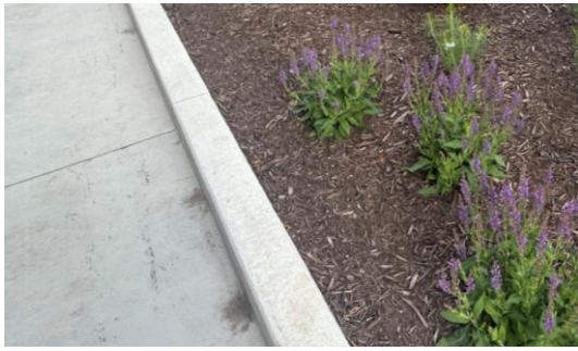
concrete planter curb – 14 TH
