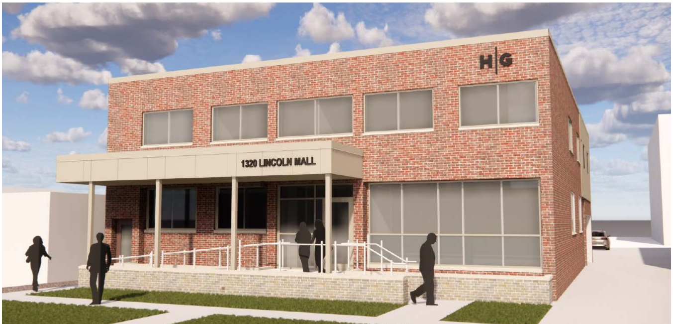
The above rendering shows the proposed improvements to the south façade for 1320 Lincoln Mall, including signage, metal coping along the roofline, new and expanded windows, an entry canopy structure, and a new ramp/stair system with a masonry veneer.
