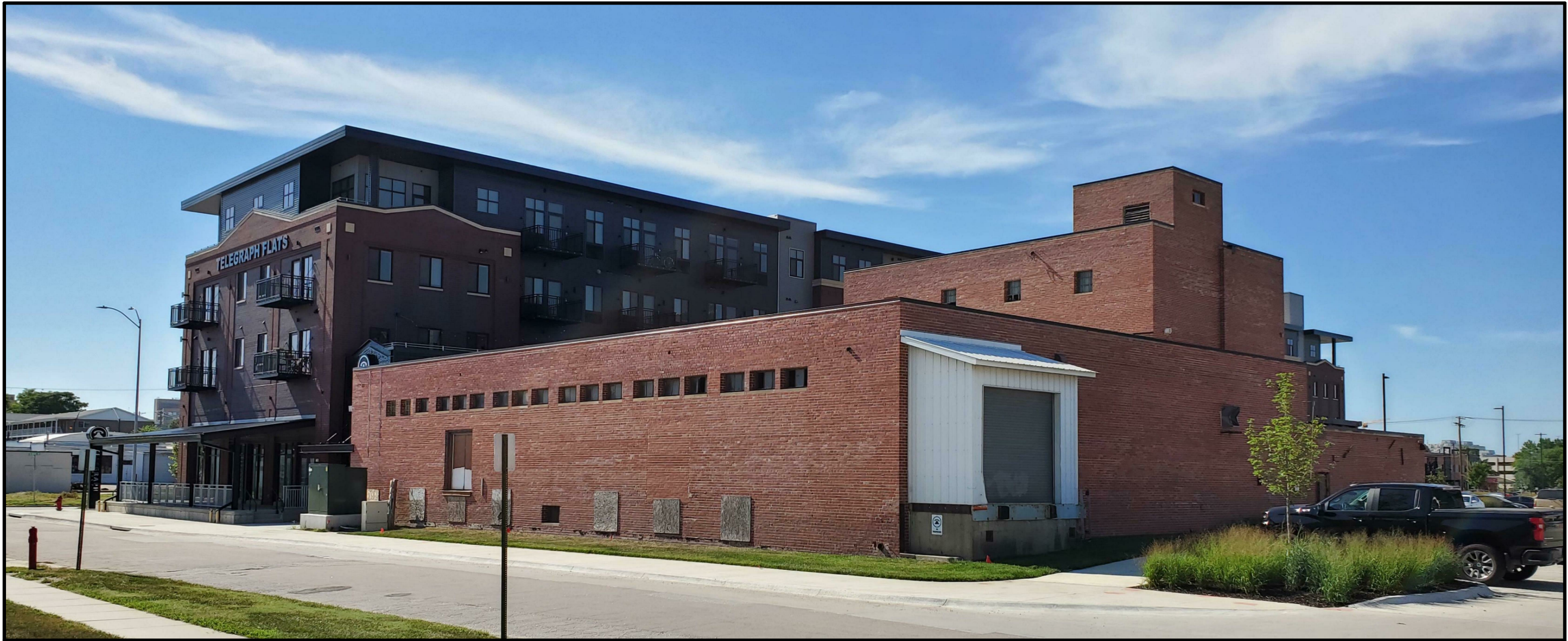
TELEGRAPH WAREHOUSE EXISTING CONDITION
