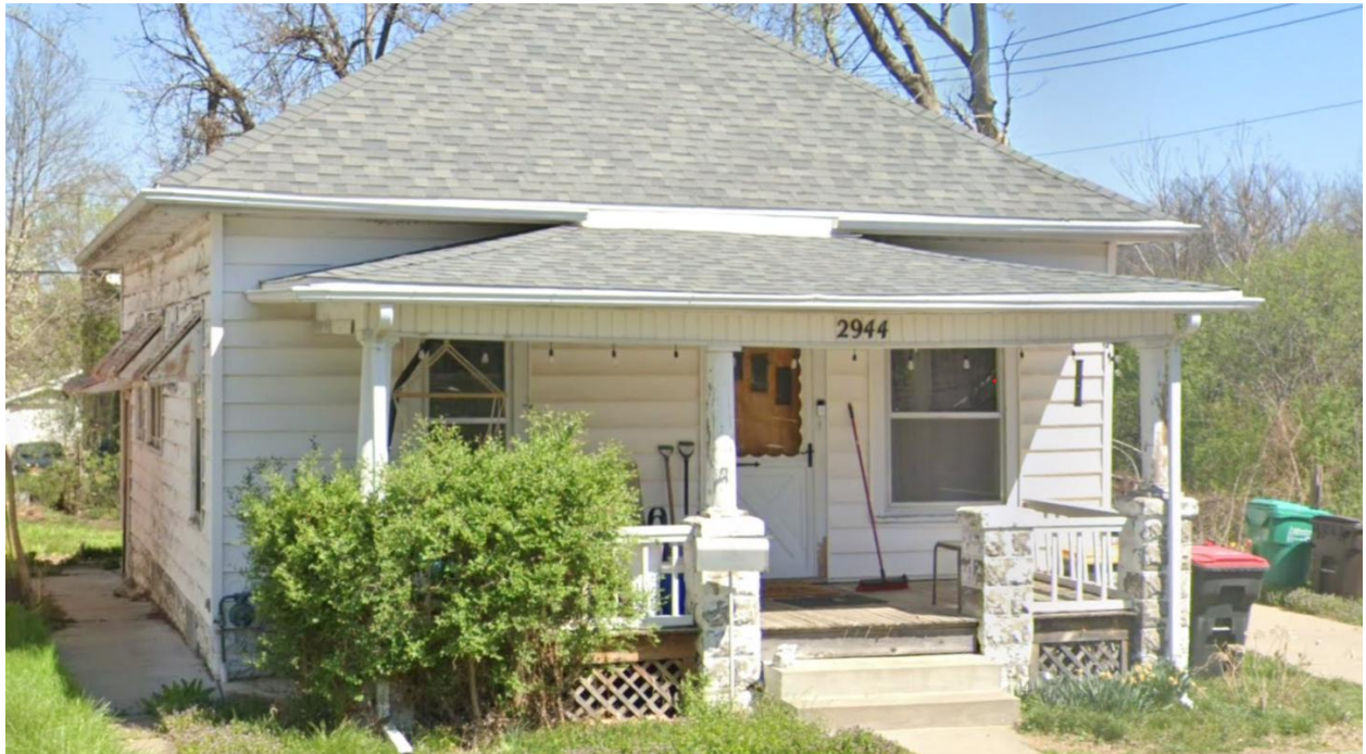
2926 Sumner Street – Front Canopy Overhang roughly 3:12 to 4:12 pitch
