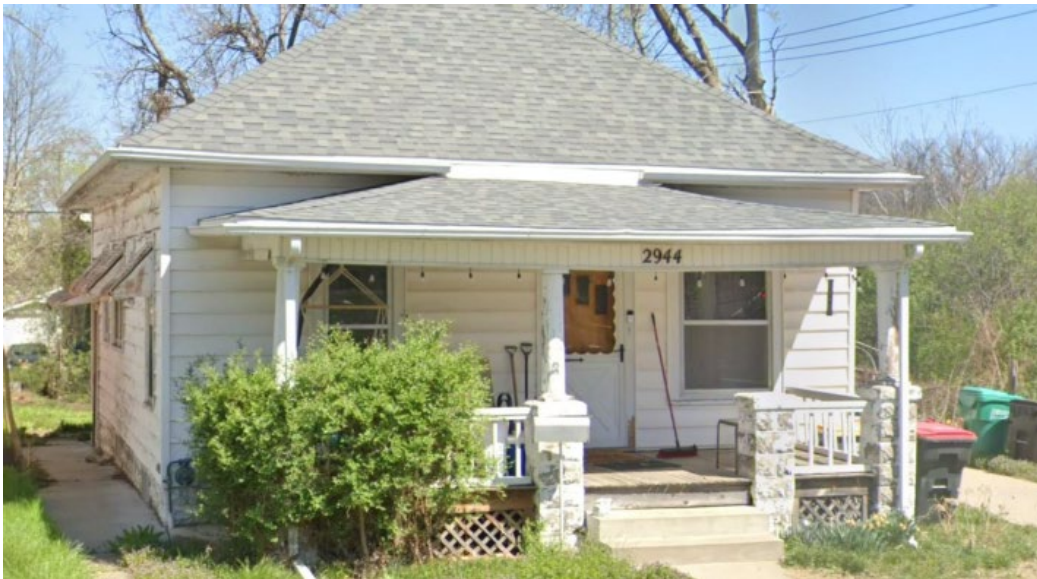
Figure 1 2944 Sumner Street, front porch with 3:12 to 3.5:12 pitch
