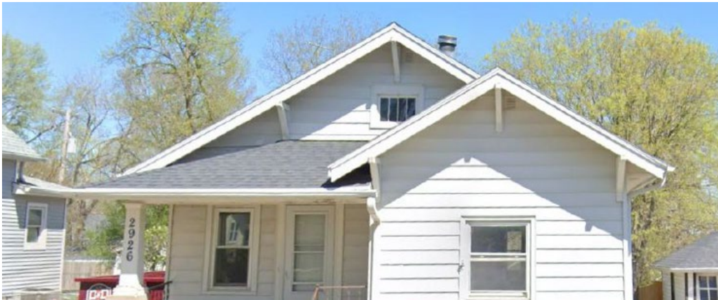
Figure 2 2926 Sumner Street, front canopy overhang roughly 3:12 to 4:12 pitch
