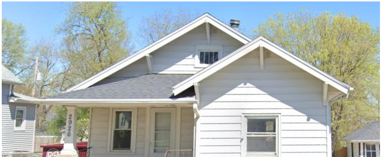
2926 Sumner Street – Front Canopy Overhang roughly 3:12 to 4:12 pitch
