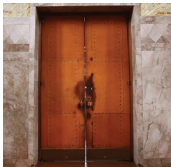
The 9-foot Library doors were renovated. The exterior with walnut and the interior with pigskin and bronze studs. Staff also created new handles to better protect the leather.
