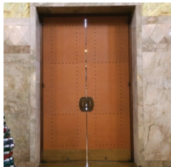
The 9-foot Library doors were renovated. The exterior with walnut and the interior with pigskin and bronze studs. Staff also created new handles to better protect the leather.
