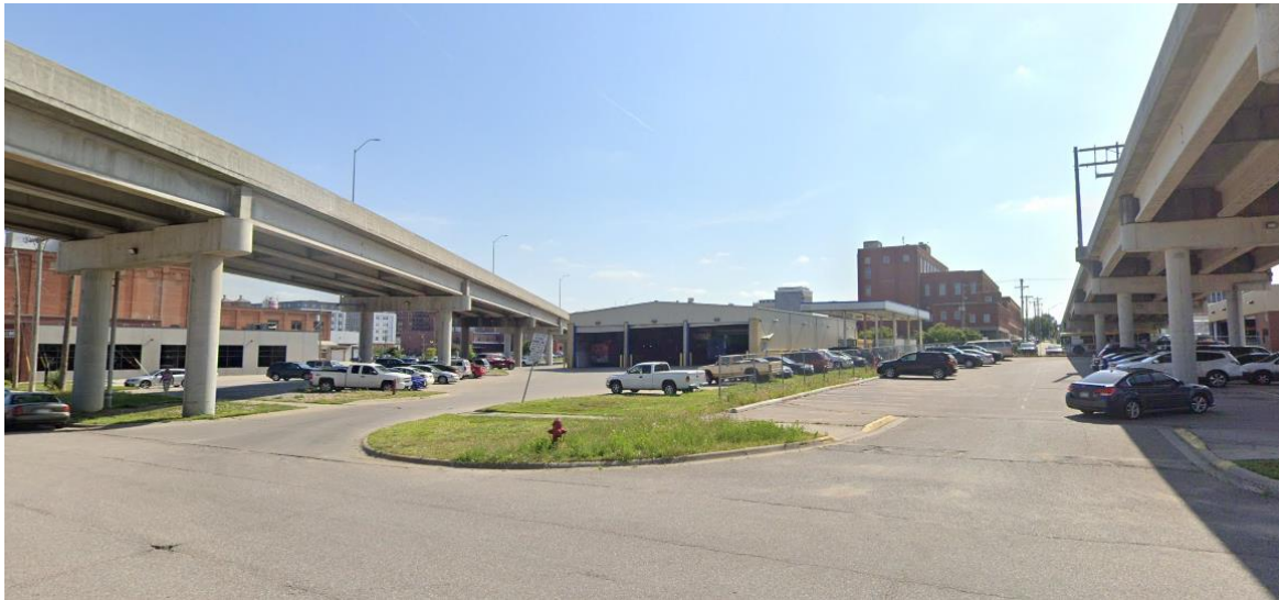
View from 7 th Street looking East
