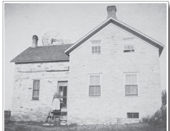
The Krull house was built in the 1860s in Lancaster County between Roca and Sprague.
