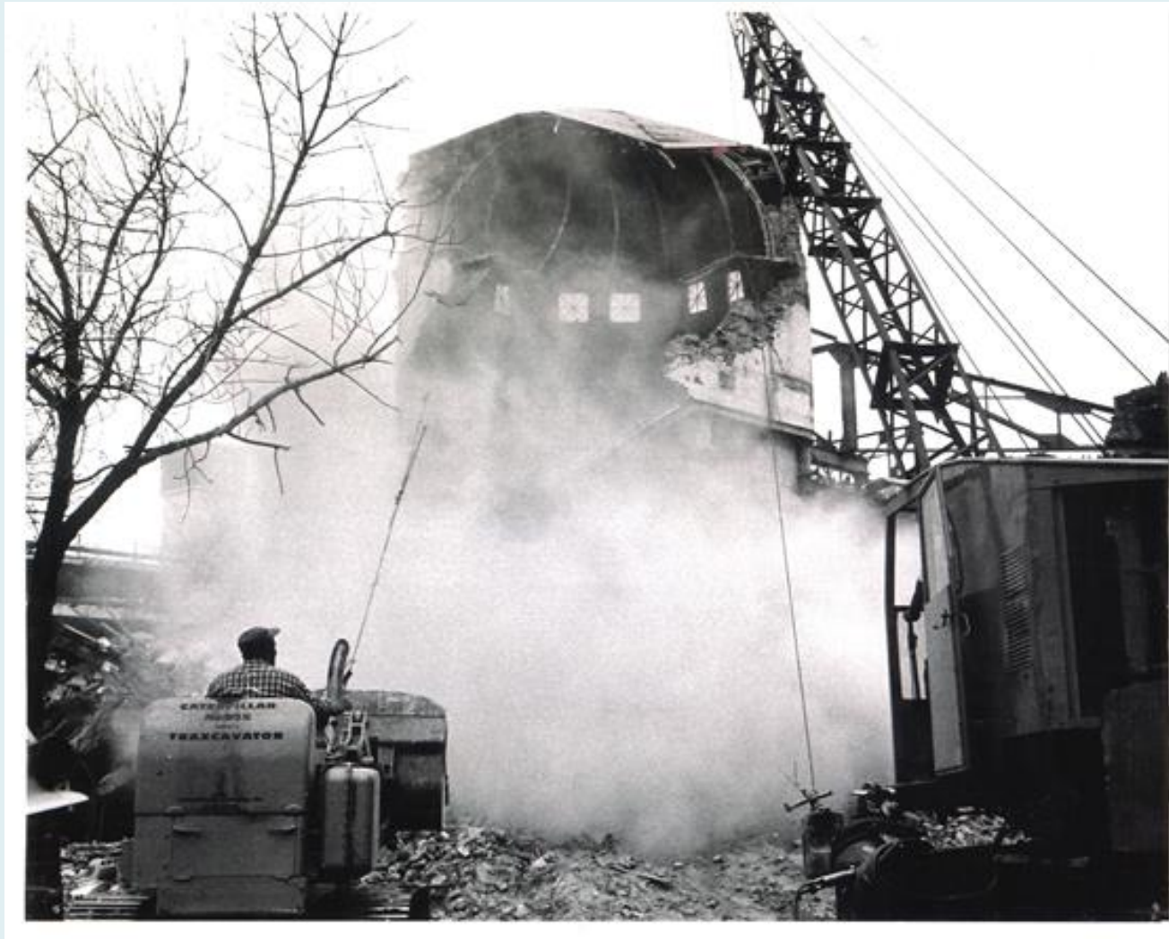
Demolition of Old Main in 1961
