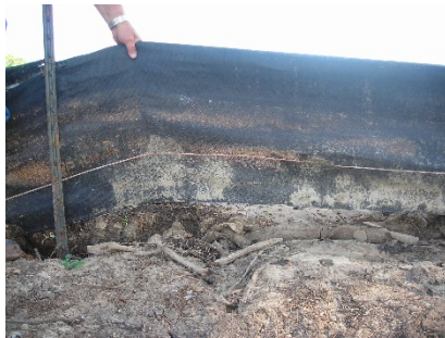
Failed Silt Fence Inspection
