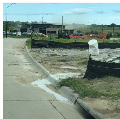
Illicit Discharge entering Storm Drain
