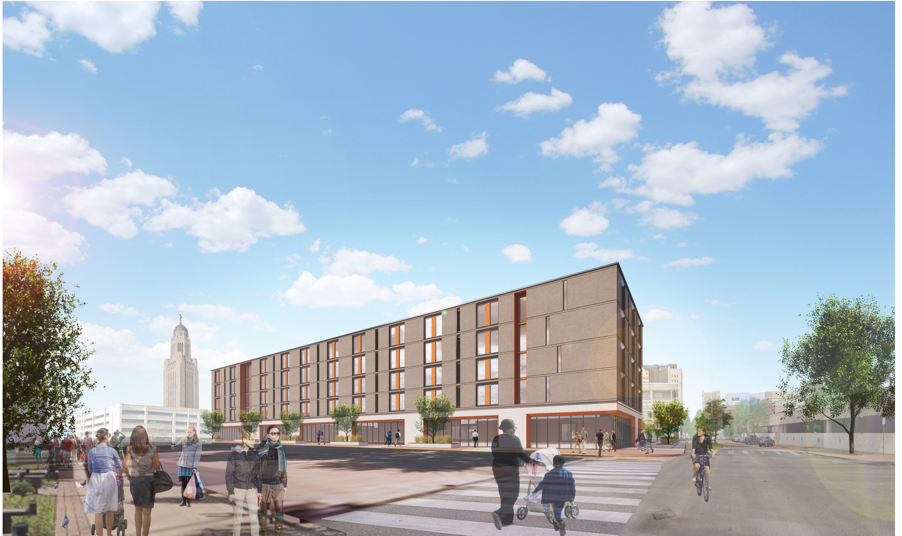
VIEW NORTHEAST CORNER
