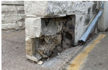
North Side Retaining Wall
