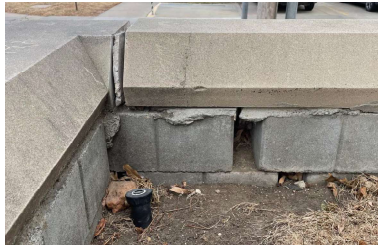
West Retaining Wall (Back Side)
