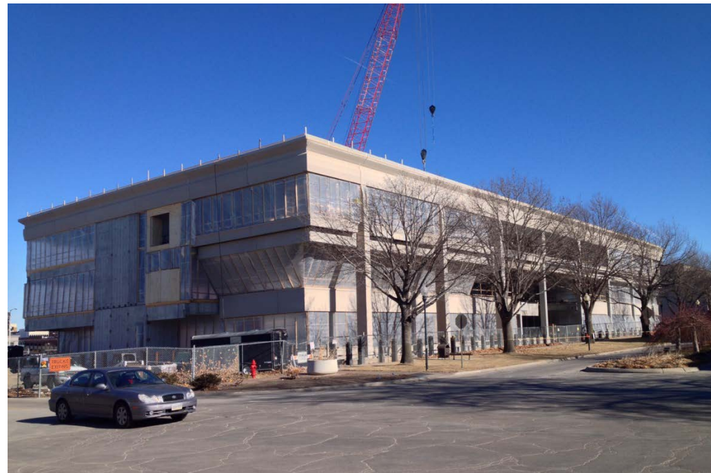
Photo of Construction Progress, Fall 2013
