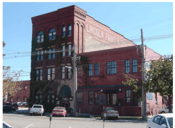
Lincoln Paint and Color Co. Building, "Color Court"
